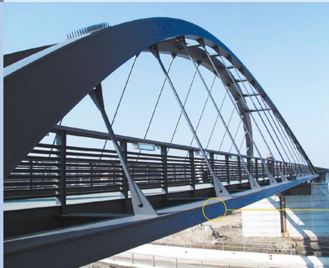
Bridge – Berlin, Germany
